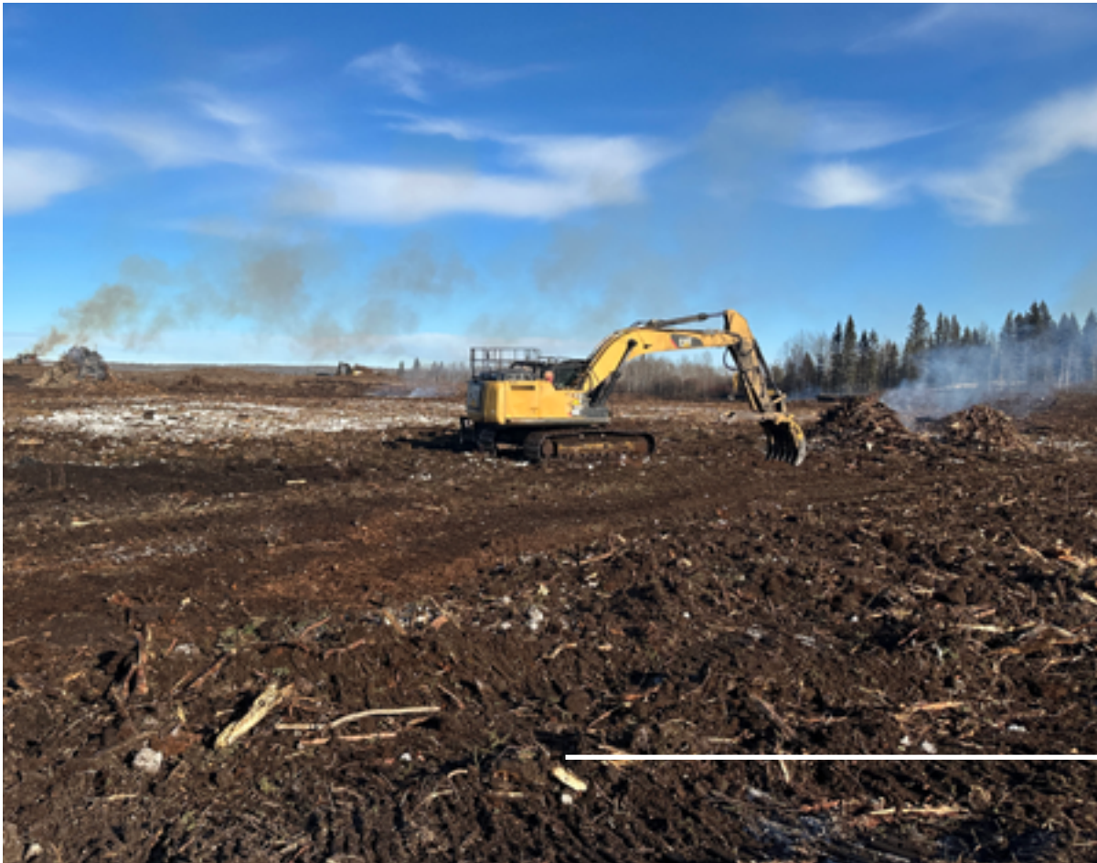
An excavator works within the Kikino Metis Settlement Community Fireguard project area
