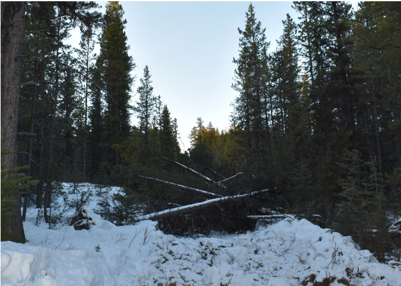
Tapper Access "Go-Around" – full line blocking was used, but trapper access was ensured through the adjacent stand.
