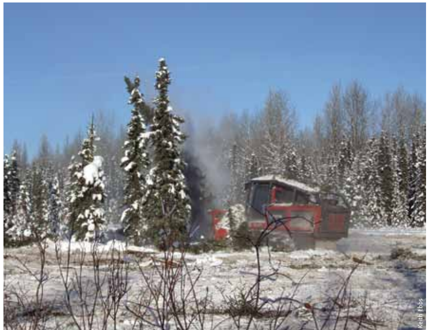
A mulcher engaged in FireSmart work in west-central Alberta
